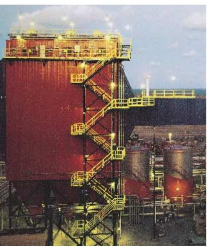
Seawater-based flue-gas desulphurisation plant
