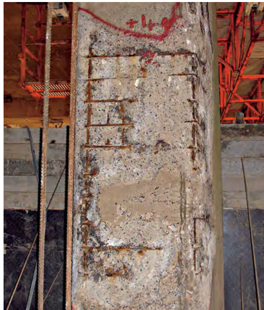
The maritime environment had taken a toll on the mosque's ocean-front portions, leading to deterioration of the pillars under the prayer room. Photo: Ugitech.
