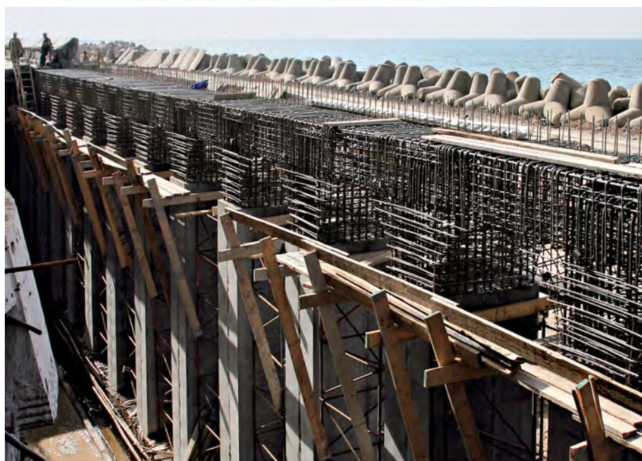
100 external “combs” supporting the peripheral slabs were rebuilt with high-performance concrete-reinforced stainless steel rebars (2205 duplex) to ensure a long lifespan for the sacred building. Photo: Ugitech.
