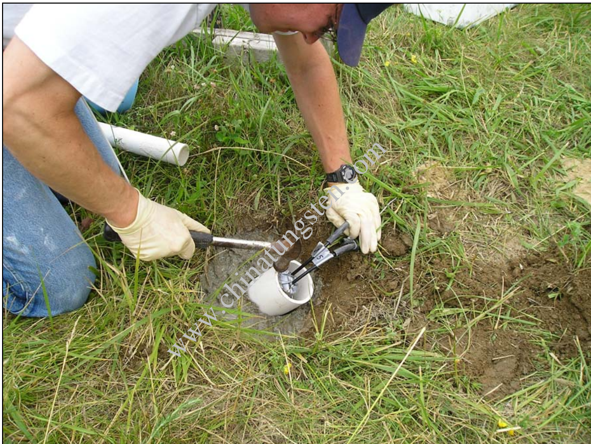
Figure A-5. Tension lysimeter installation.
